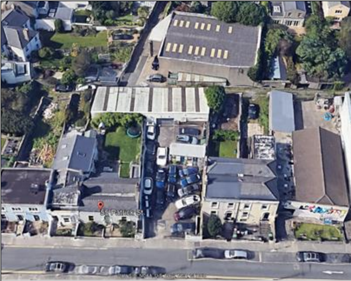
Fig. 1.0 – Aerial view of site
